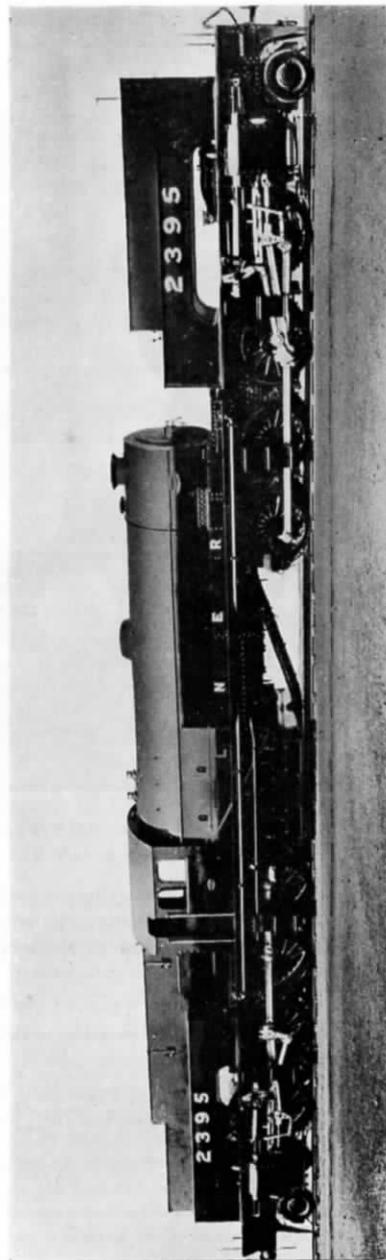
FIG. 267.—SIX-CYLINDER GARRATT LOCOMOTIVE 2-8-0+0-8-2 TYPE, L.N.E.R.
