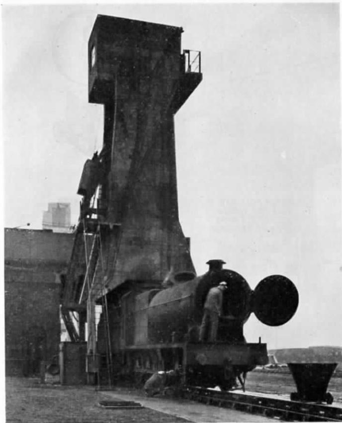
FIG. 16.—NARROW-GAUGE TROLLEY FOR REMOVING ASHES FROM SMOKEBOX AND ASHPAN.
