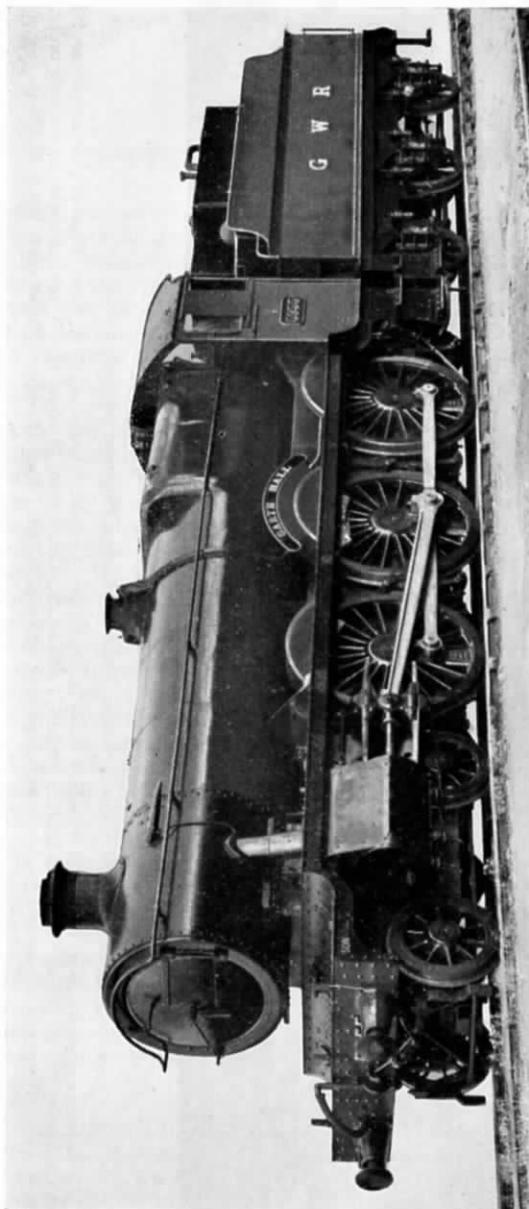
FIG. 27.—4-6-0 LOCOMOTIVE No. 5955, "GARTH HALL," G.W.R., CONVERTED TO OIL BURNING. THE TANKS FOR THE LIQUID FUEL CAN BE SEEN ON THE TENDER.
