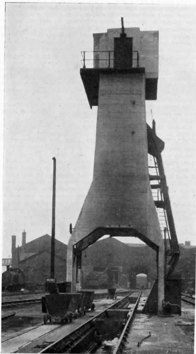
FIG. 17.—COALING AND ASH PLANT AT KENTISH TOWN, L.M.S.R.
