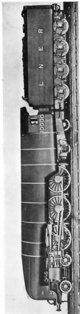
FIG. 285.—L.N.E.R. ENGINE No. 10000 AS ORIGINALLY BUILT IN 1929, FOUR-CYLINDER COMPOUND ;
