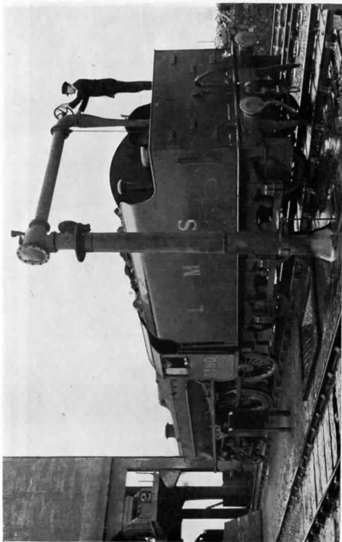
FIG. 177.—COALING AND WATERING A LOCOMOTIVE TENDER UNDER MODERN CONDITIONS.
