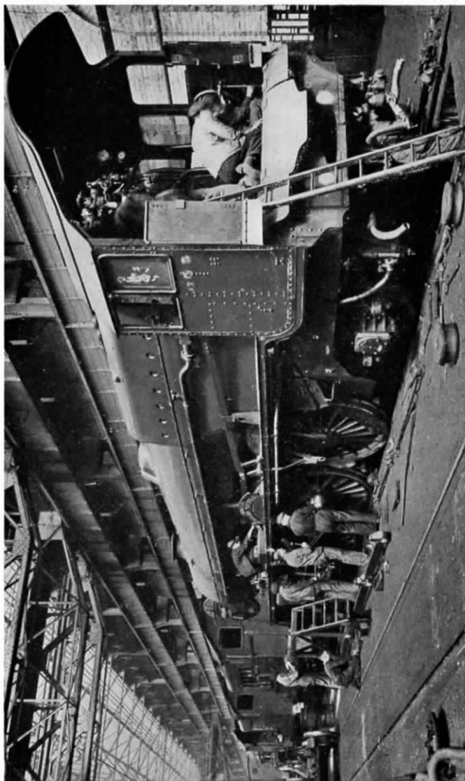
FIG. 63.—VIEW IN THE ERECTING SHOP AT CREWE, L.M.S.R., SHOWING 4-6-2 LOCOMOTIVE No. 6208 UNDER REPAIR.
