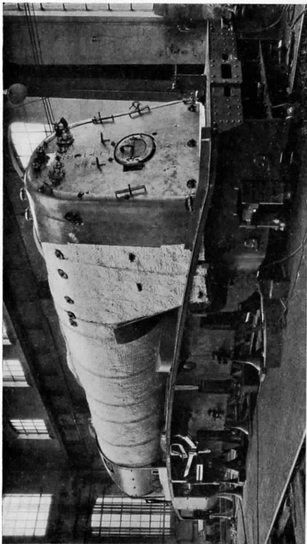
FIG. 33.—LOCOMOTIVE BOILER LAGGED WITH "ALFOL" INSULATING MATERIAL.
