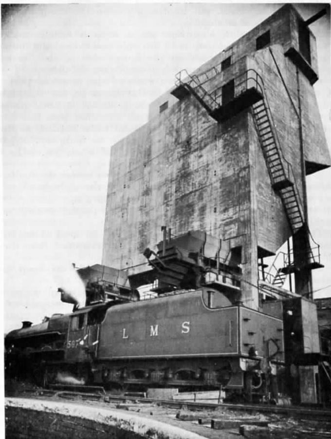
FIG. 14.—MECHANICAL LOCOMOTIVE COALING PLANT AT PRESTON, L.M.S.R.
