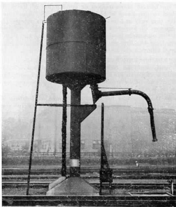
FIG. 31.—A TYPE OF WATER COLUMN INSTALLED ON THE SOUTHERN RAILWAY.
