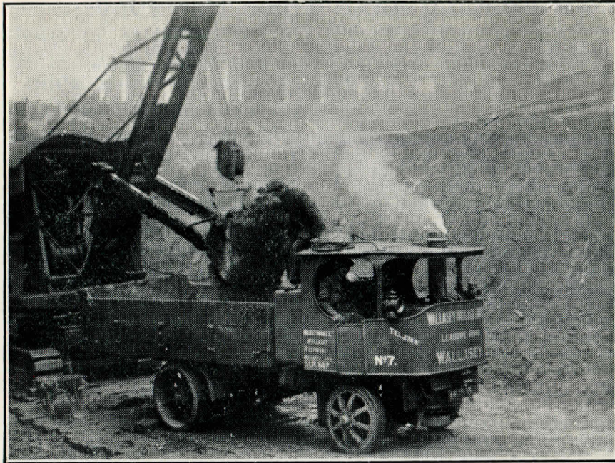
A large steam navvy, employed on the excavation work for the Woolworth building in Church Street, Liverpool, loading direct into a "Sentinel" waggon.
