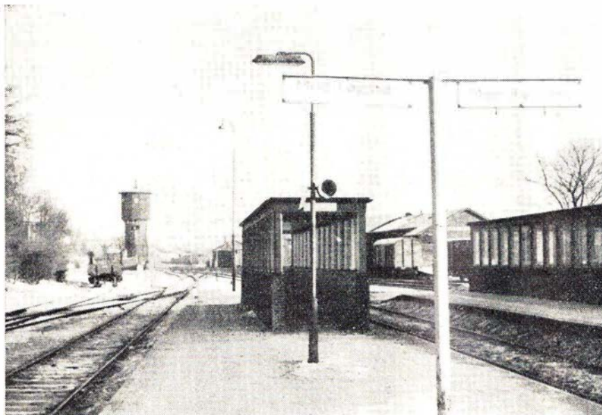
Hobro station perron 3
